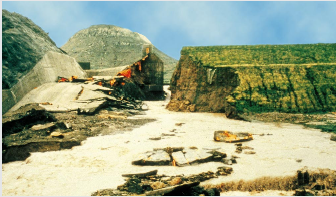
Failure of an earthfill dam in Lesotho due to internal erosion
